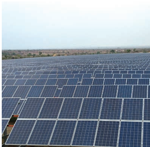
28.8 MW Palaswadi Solar Project
