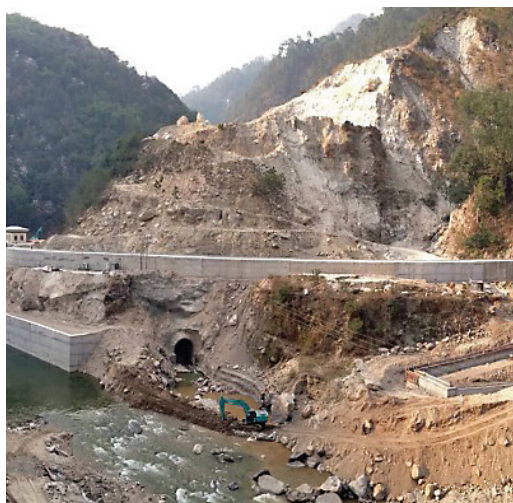
126 MW Dagachhu Hydro Project
