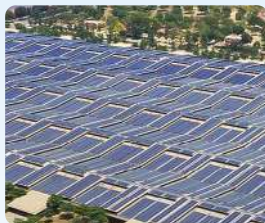
World's largest solar rooftop installation of 12 MW for RSSB-EES, Amritsar (single location, multi-roof)
