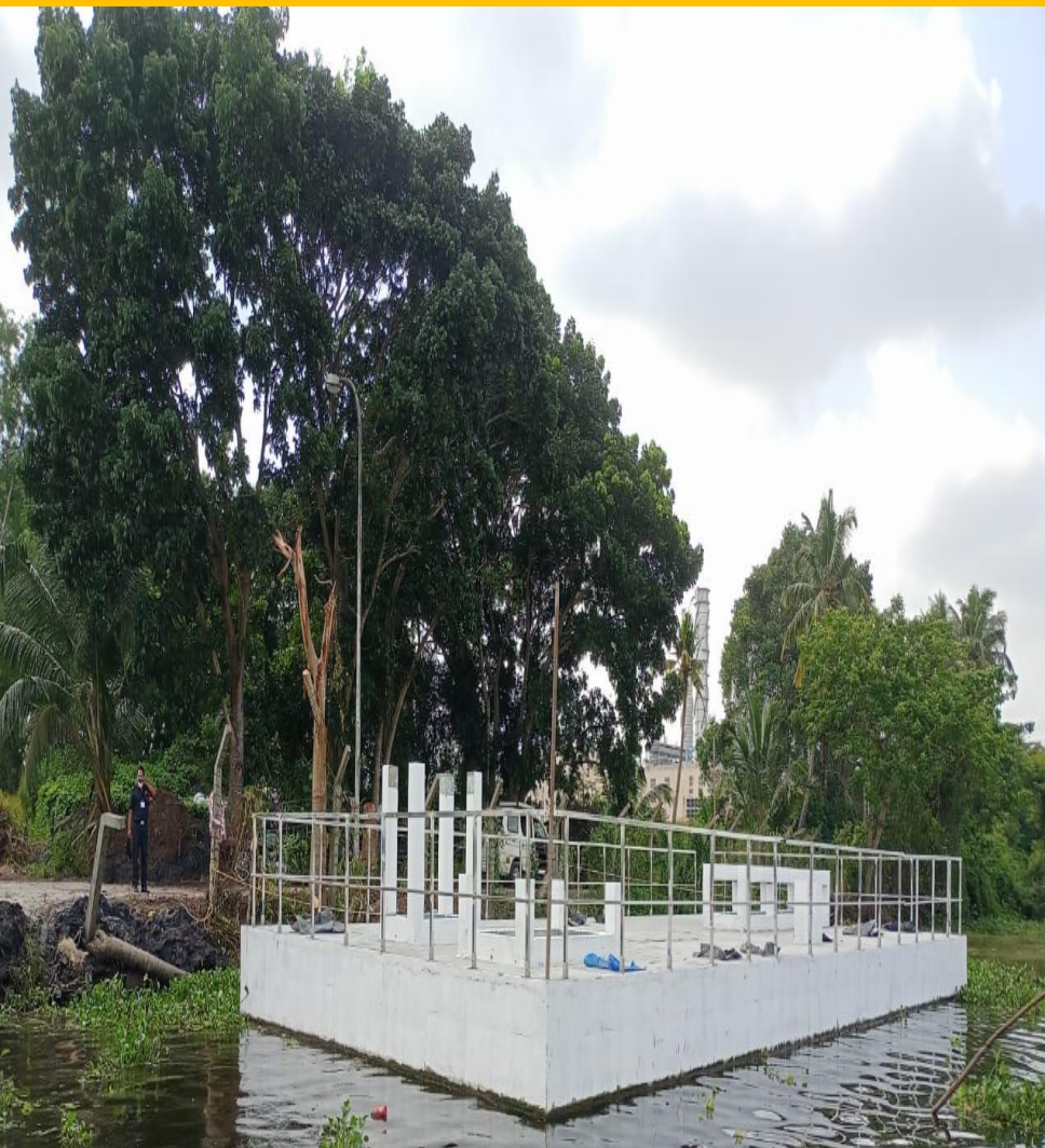
Inverter Ferro cement Platform completion
