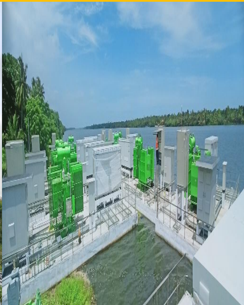
Equipment Erection on Platform
