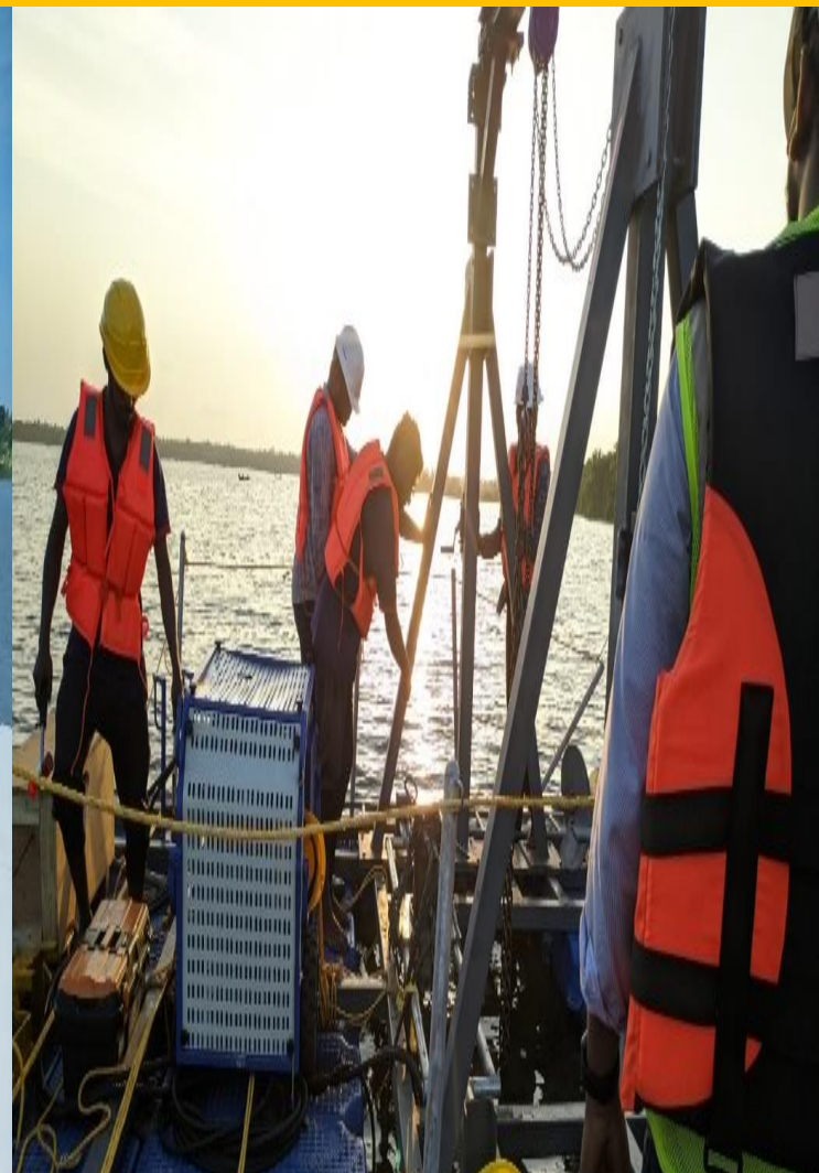
Anchoring of floater in water
