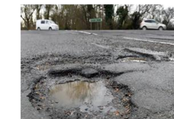
Road repair solutions
