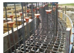
Heavily reinforced structure
