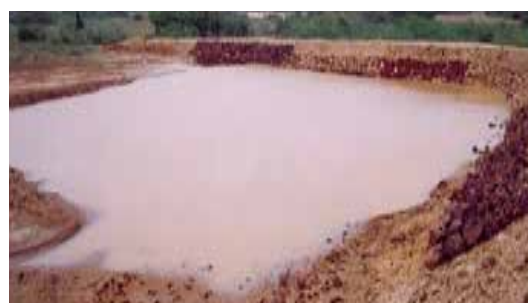
Construction of Nala Plugs
