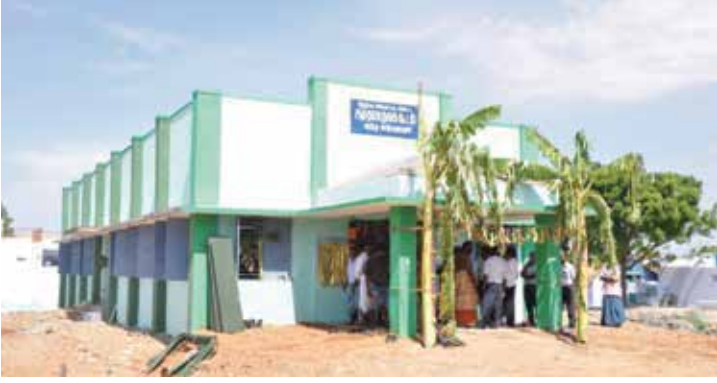
COMMUNITY HALL CONSTRUCTED FOR PEOPLE OF SEZHIANALLUR VILLAGE, SANKARNAGAR
