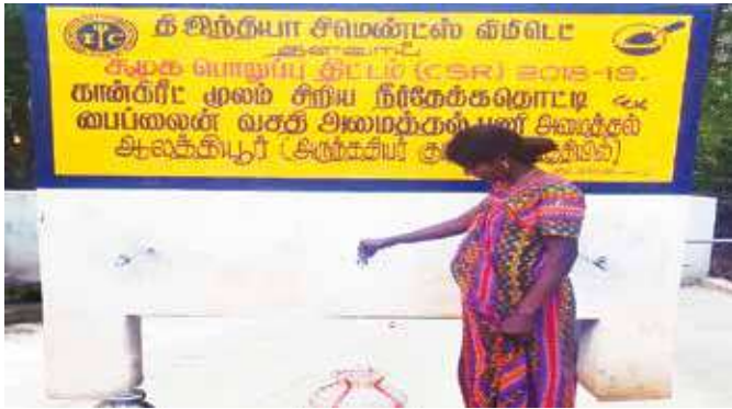
Providing drinking Water Facility to Villagers
