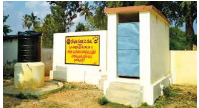
Construction of restroom at Government School
