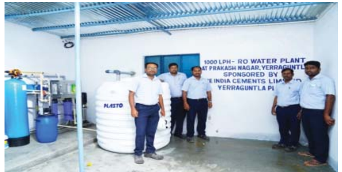
Installation of RO plant
