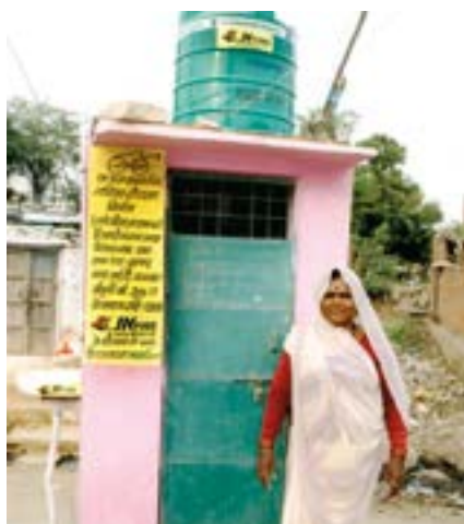
Contributing towards making India cleaner through construction of Toilets
