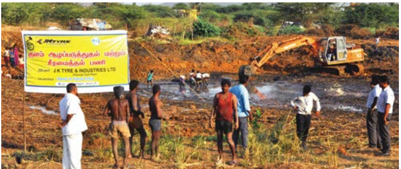
Desiltation of tanks for Water Conservation
