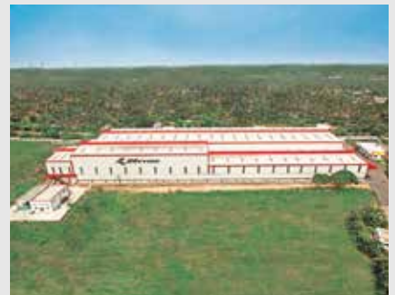
New OTR Plant in Mysuru
