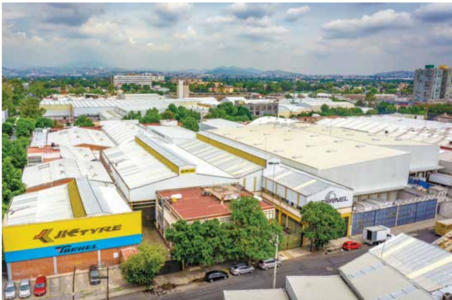
JK Tyre Tornel Plant, Mexico
