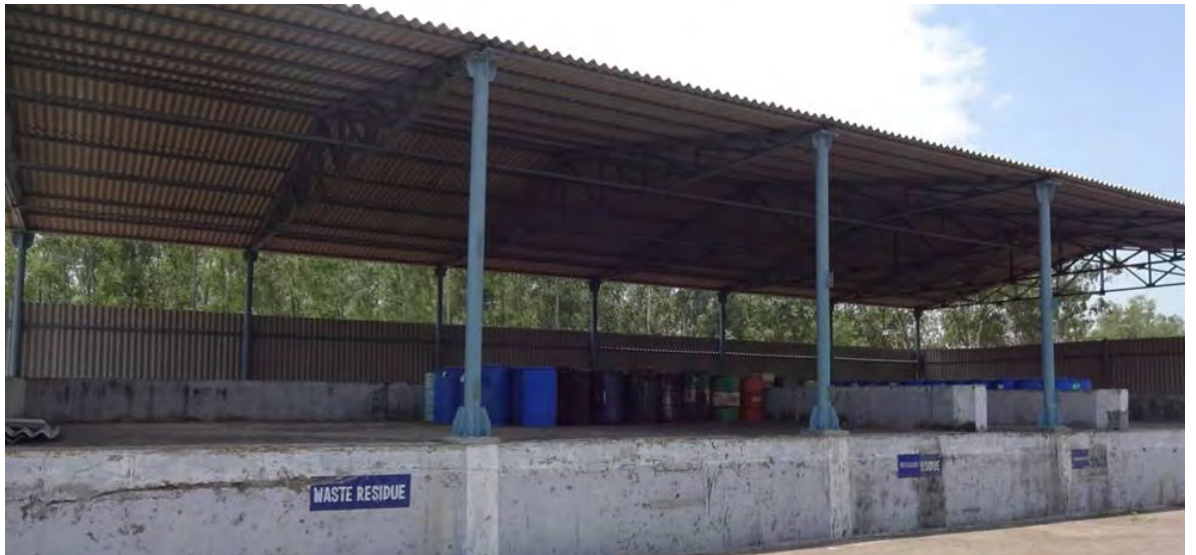
Hazardous waste storage area
