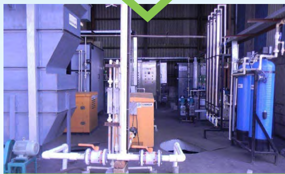
New Effluent Treatment Plant at Ambernath
