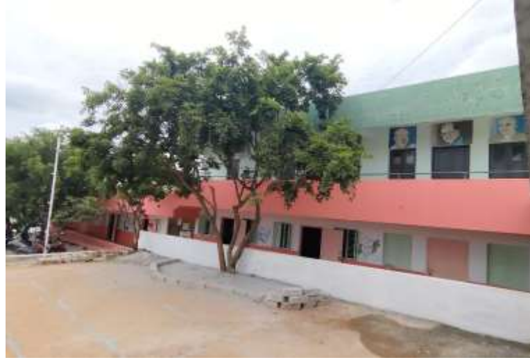
Renovation of classrooms, Uttarahalli - CKP
