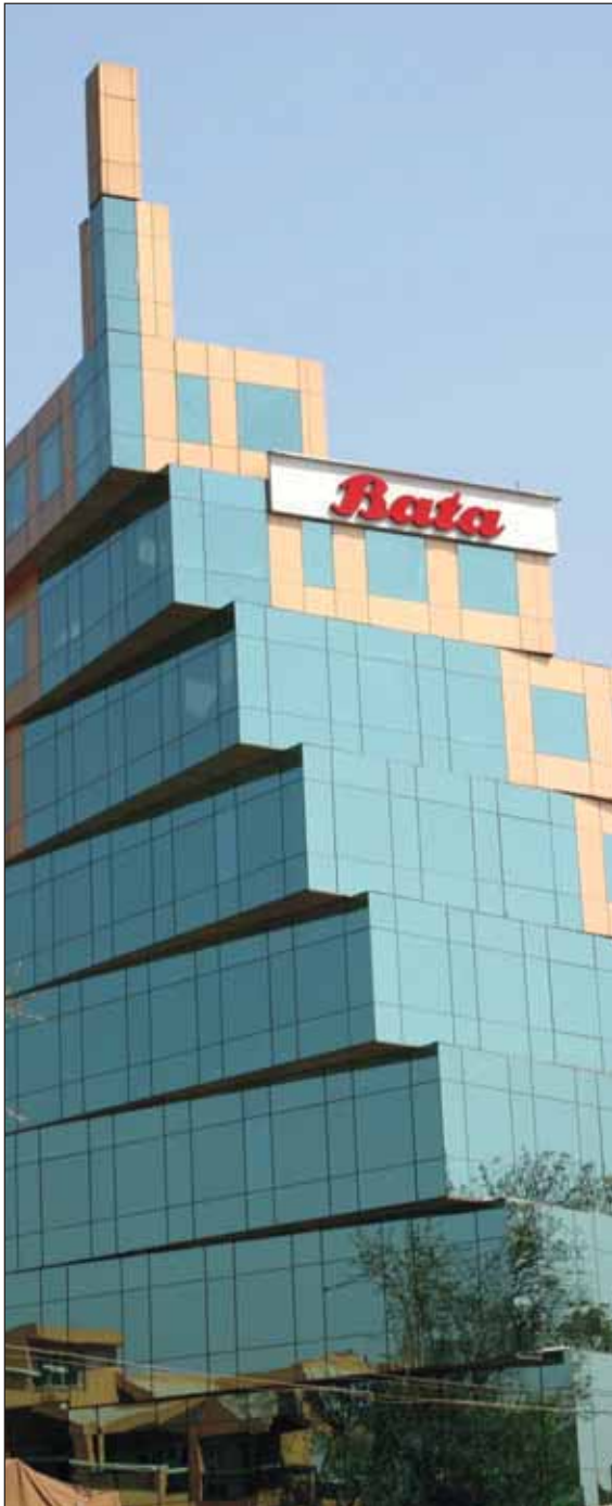
Bata India's Corporate Office At Gurgaon, Haryana
