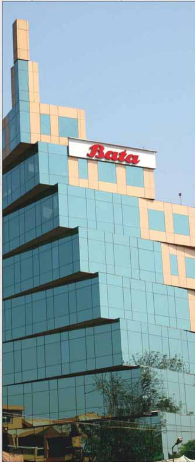
Bata India's Corporate Office At Gurgaon, Haryana
