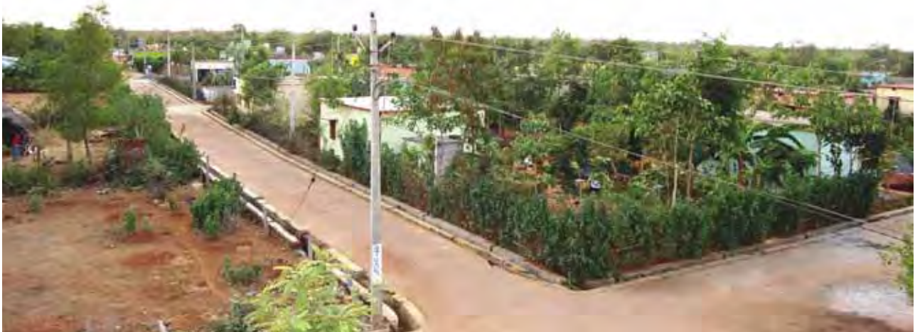
Roads, electricity and potable water are just some of the amenities that the residents of the Trijanga township enjoy.
