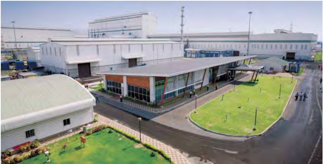
The Tata BlueScope Steel facility at Bara, Jamshedpur.
