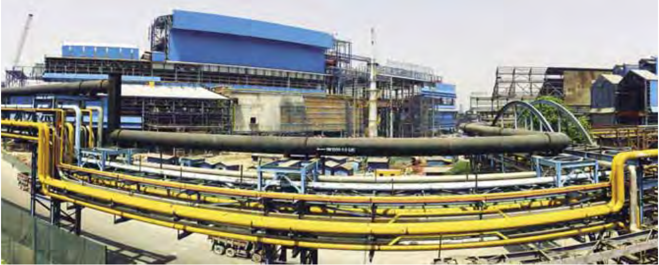
Site of the 2.9 mtpa expansion at Jamshedpur.
