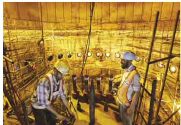
The inner shell of the new I Blast Furnace at Jamshedpur.
