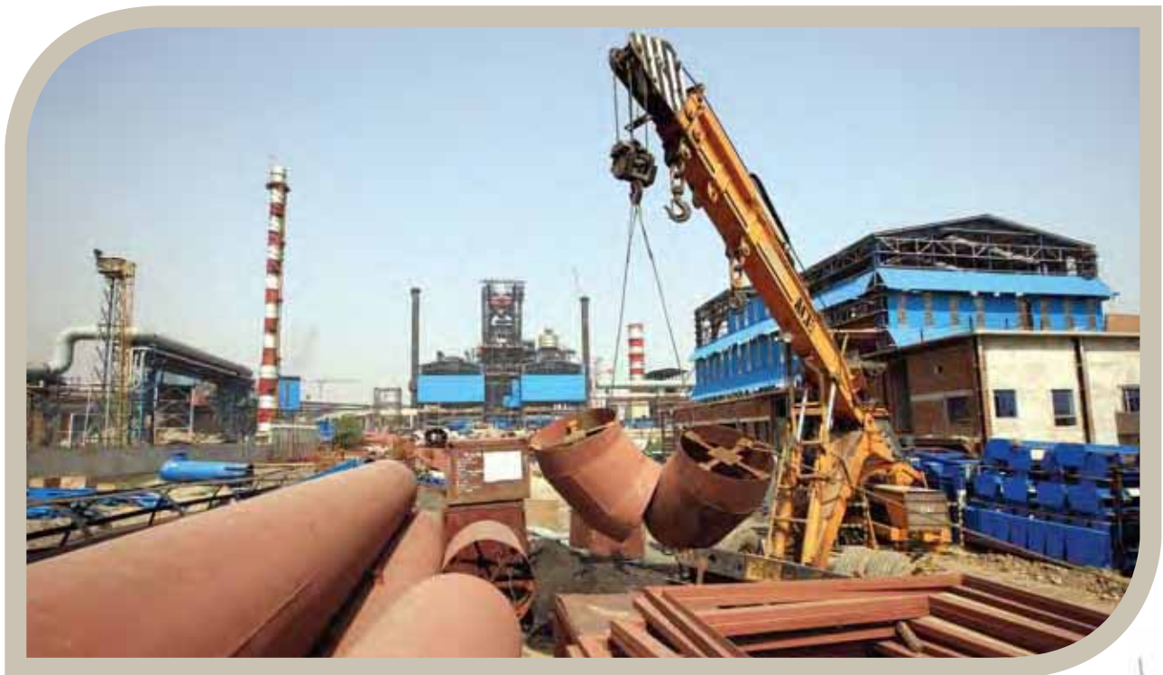
Brownfield expansion at Jamshedpur, India
