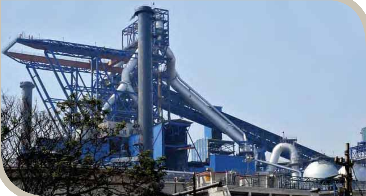
Brownfield expansion "I" Blast furnace, Jamshedpur, India
