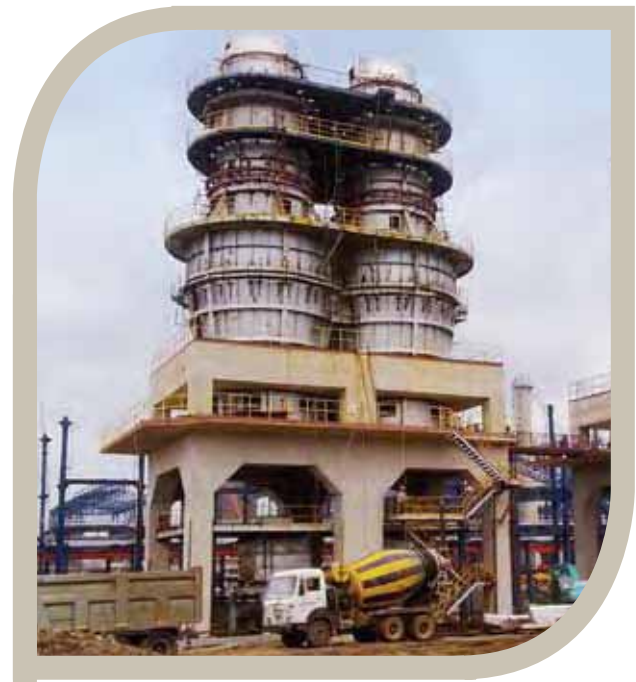
Greenfield project – Kiln 2, Odisha, India
