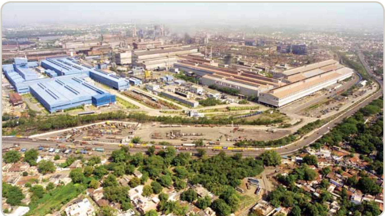
Pan-view of facility in Jamshedpur, India
