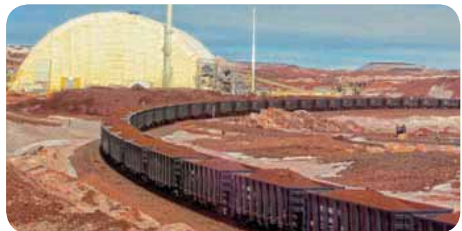
Processing facilities and Rail Loop
