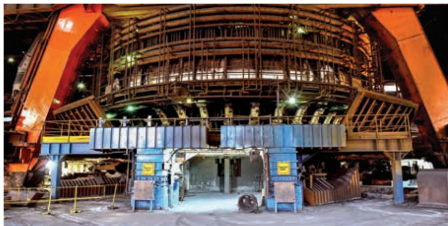
Resource-efficient blast furnaces with high productivity
