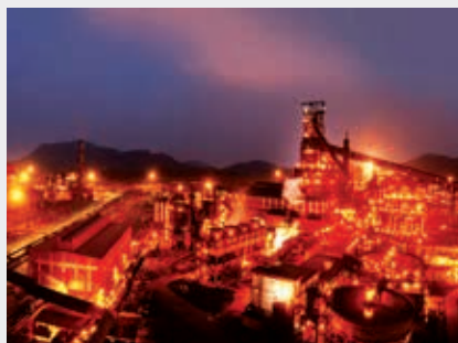
Capacity Expansion at State-of-the-art Kalinganagar Steel Plant
