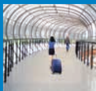
iGATE Skywalk in Bengaluru
