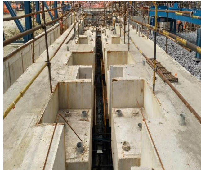
PLTCM equipment foundation
