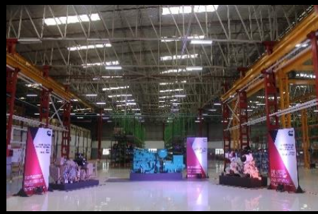
Power Systems Plant, Pirangut 2018
