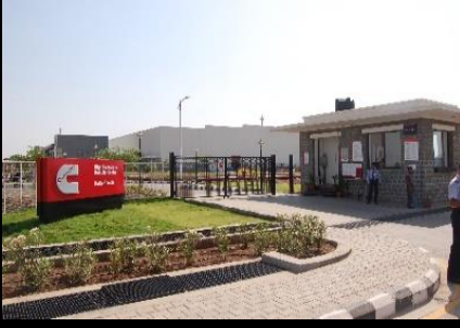
HHP Rebuild Center 2011
