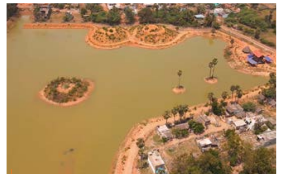
Eco-restoration of Nagan Thangal lake in Chennai, Tamil Nadu as part of Project Nanneer
