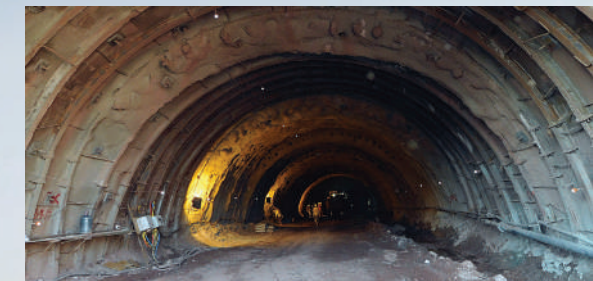
Udhampur-Srinagar-Baramullah Rail Link - T15, Jammu & Kashmir
