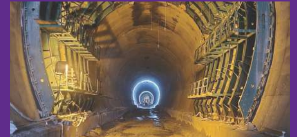
Kiru Hydroelectric Project, Jammu & Kashmir
