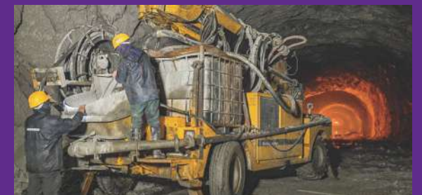
Luhri Hydroelectric Project, Himachal Pradesh
