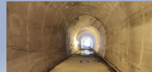
Udhampur-Srinagar-Baramullah Rail Link - T2, Jammu & Kashmir
