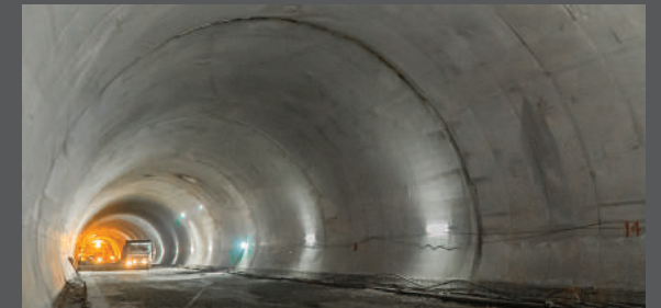
Sela Road Tunnel, Arunachal Pradesh
