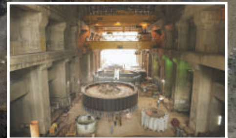
Subansiri Hydroelectric Project, Assam
