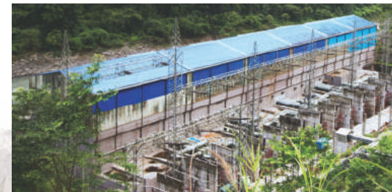
Kimi Sub Surface Power House (Kameng HEP), Arunachal Pradesh
