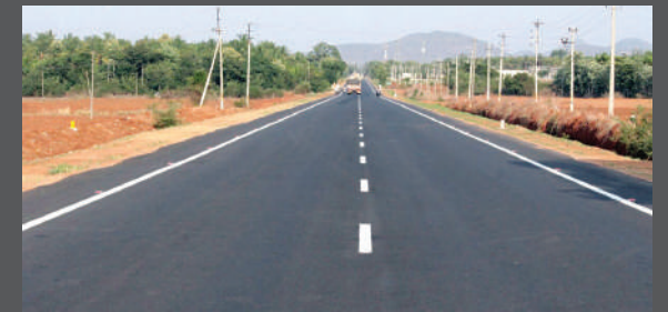
Shimoga Highway, Karnataka
