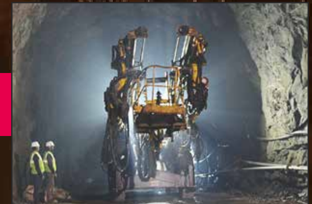
Kundah Hydroelectric Project, Tamil Nadu
