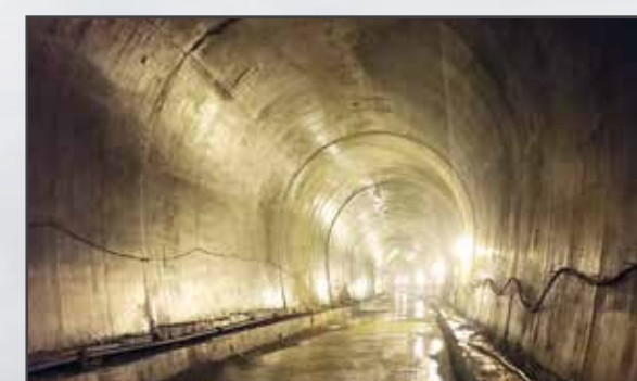
Udhampur-Srinagar-Baramullah Rail Link - T2, Jammu & Kashmir
