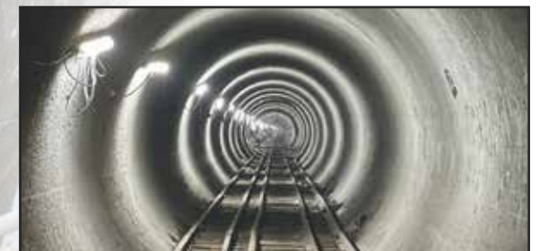
AMT-2 Water Supply Project, Maharashtra
