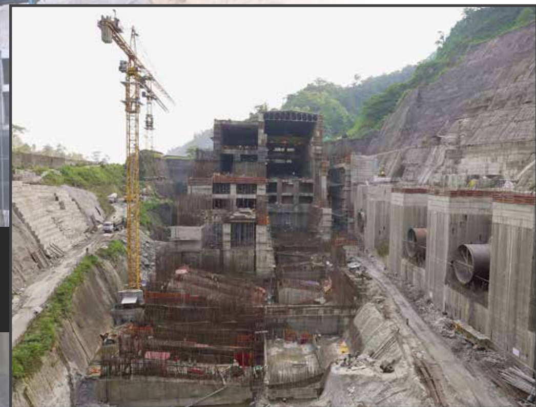
Subansiri Hydroelectric Project, Assam
