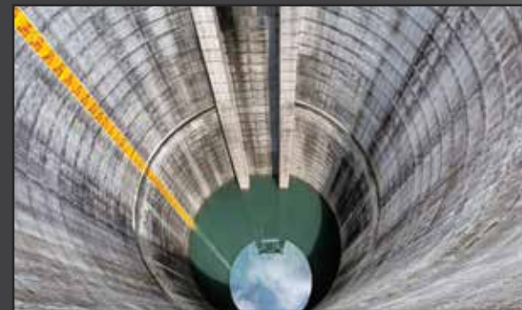
Rampur HEP, Himachal Pradesh
