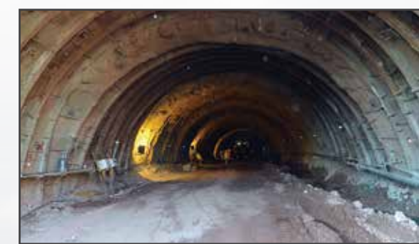
Udhampur-Srinagar-Baramullah Rail Link - T15, Jammu & Kashmir
