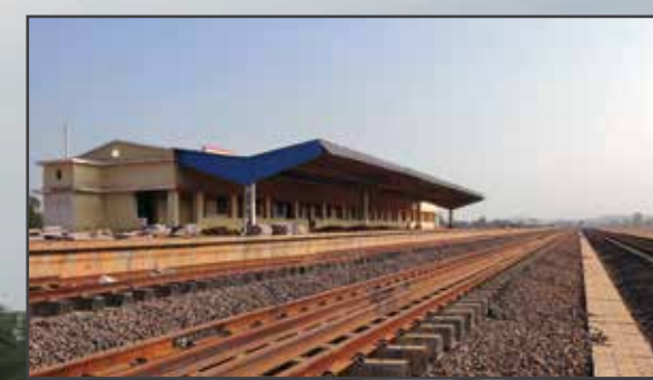
RVNL - KTR Rail Project, Chhattisgarh
