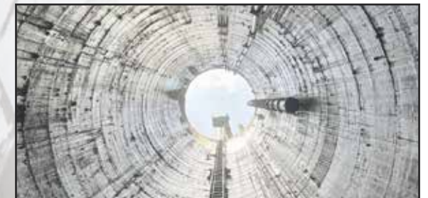
PGRW Water Supply Project, Maharashtra
