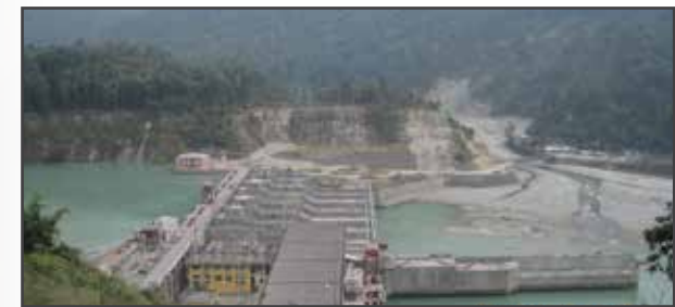
Teesta Barrage, West Bengal
