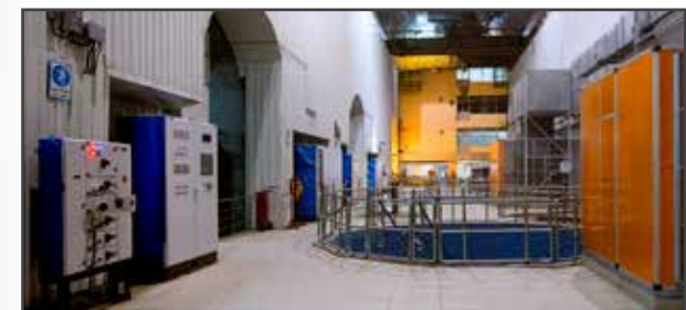
Sawrakuddu Underground Power House, Himachal Pradesh
