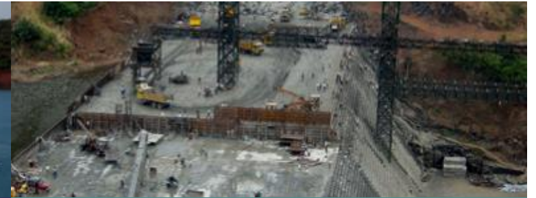
Roller Compacted Concrete (RCC)
