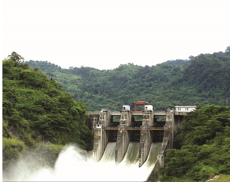
Tuirial Hydro Electro Project Mizoram (60 MW)
