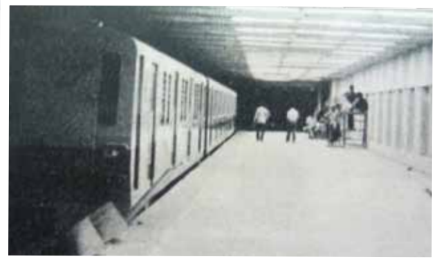
Underground air conditioning & ventilation for India's first Metro Rail in Kolkata – three stations including Park Street, the longest.
