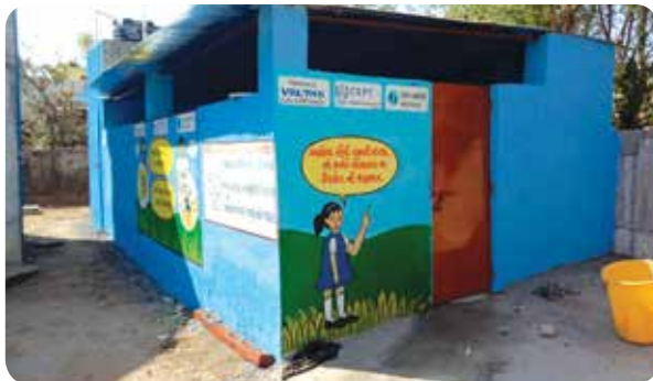
Waghodiya Kanya school urinal after intervention
