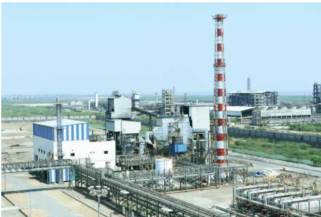
Nitric Acid plant at Dahej
