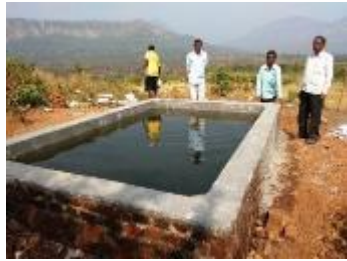
Support for water resource development and conveyance
