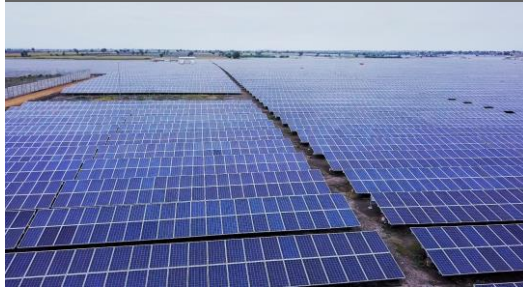
100 MW (AC) Solar Plant
