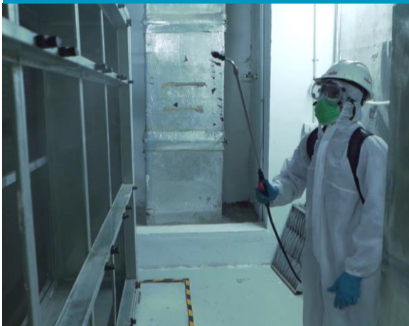
Enhanced AHU Cleaning
