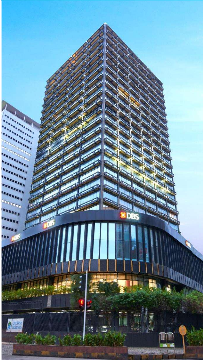
Express Towers Mumbai (0.5 msf)
