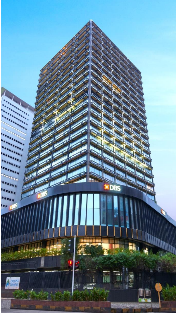
Express Towers Mumbai (0.5 msf)
