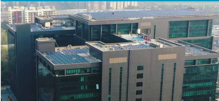
525 kW Solar Roof top at Embassy 247, Mumbai (Awarded 'Best Green Building Project of the Year')
