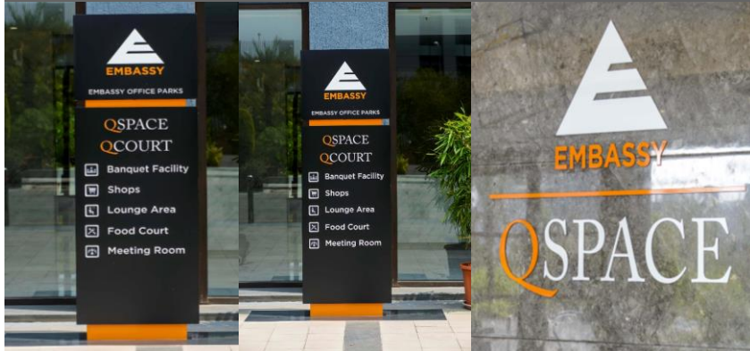
Embassy Qubix – Signage & branding upgrade (WIP, targeting Dec'19 completion)
