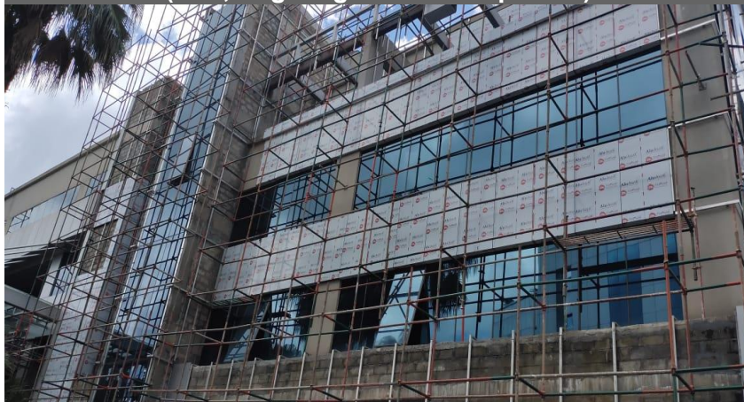
Embassy Golflinks – Crystal Down Refurbishment (WIP, targeting Mar'20 completion)
