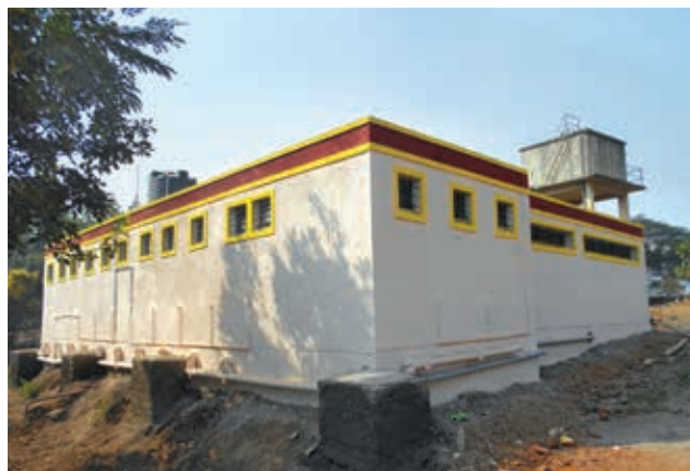
Completed sanitation unit in Maharashtra
