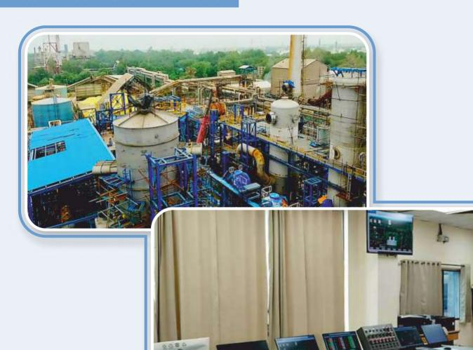
600 MTPD Sulphuric Acid-V (SA-V) Project, which has been conceptualized to meet the increasing raw material requirements for GSFC's expanding product basket. In addition, the project is designed to optimize the steam network of the complex, with steam being generated as a by-product. This will contribute to a reduction in Natural Gas consumption for steam production and accordingly it will reduce the overall energy cost.
