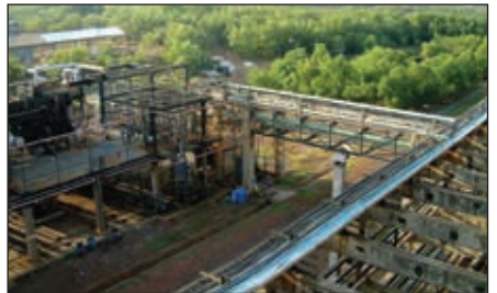
Trees planted in the Company premises
