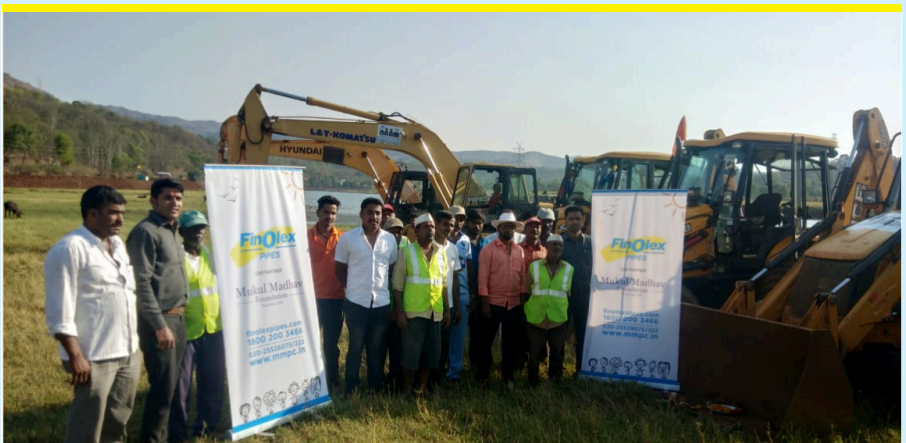
Water project at Kadakwasala, Pune District, Maharashtra
