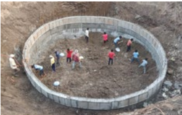
Construction of well and support of pipeline for water project in Latur for those affected by HIV.
