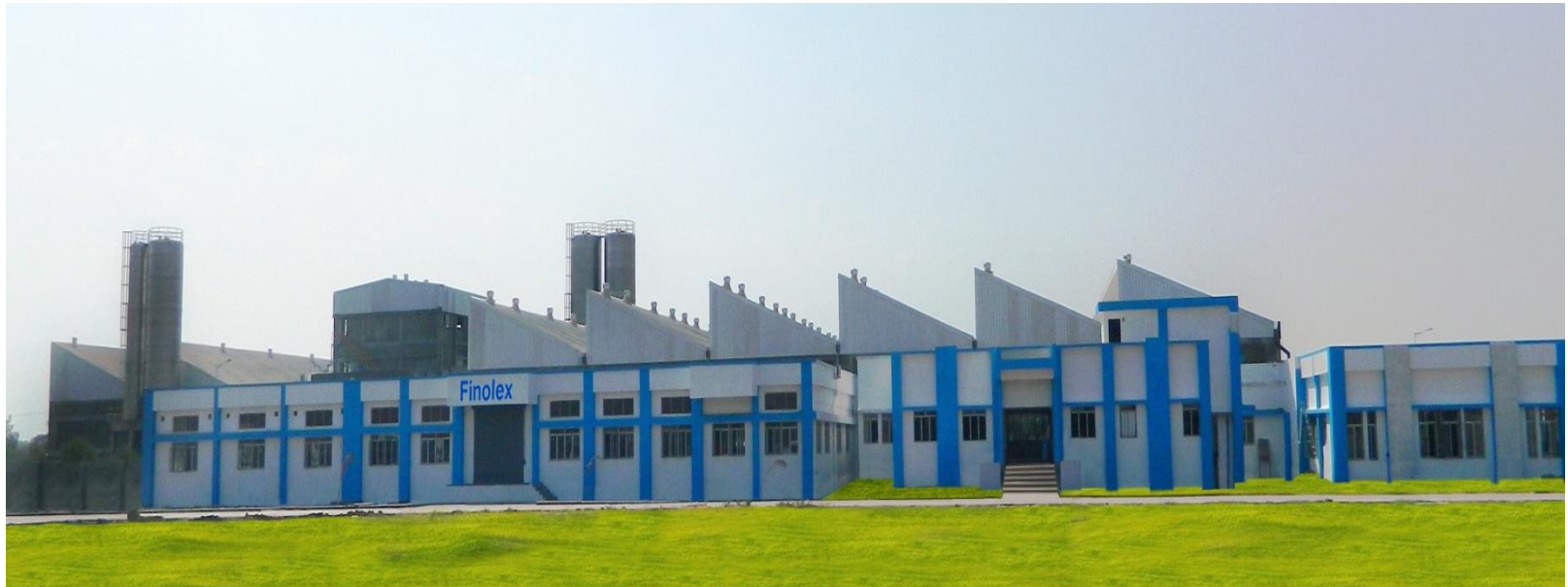
Well designed state-of-the-art infrastructure at Masar, Gujarat
