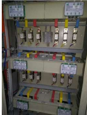
LT APFC and RTPFC panels HT APFC and Fixed Capacitor Panels
