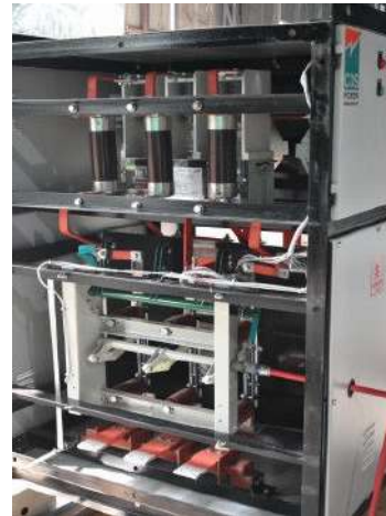
LT APFC and RTPFC panels HT APFC and Fixed Capacitor Panels
