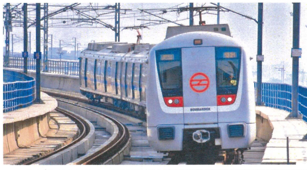
Power Quality pilot project for metro rail
