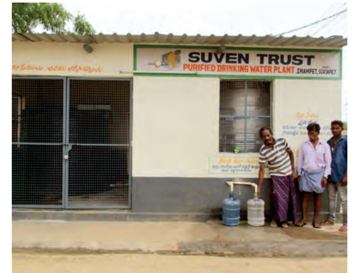
RO DRINKING WATER FACILITY AROUND SURYAPET DISTRICT IN TELANGANA
