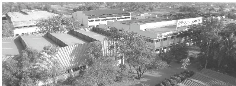
Menon Pistons Ltd. main manufacturing facility at Kolhapur.
