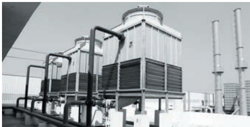
Chilling plant cooling towers
