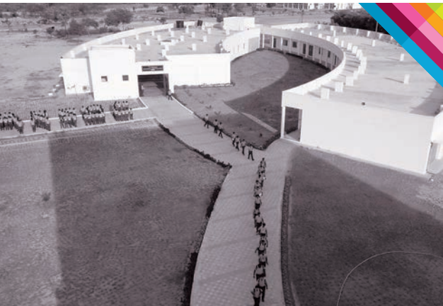
ARIEL VIEW OF THE AMARA RAJA SKILL DEVELOPMENT CENTRE
