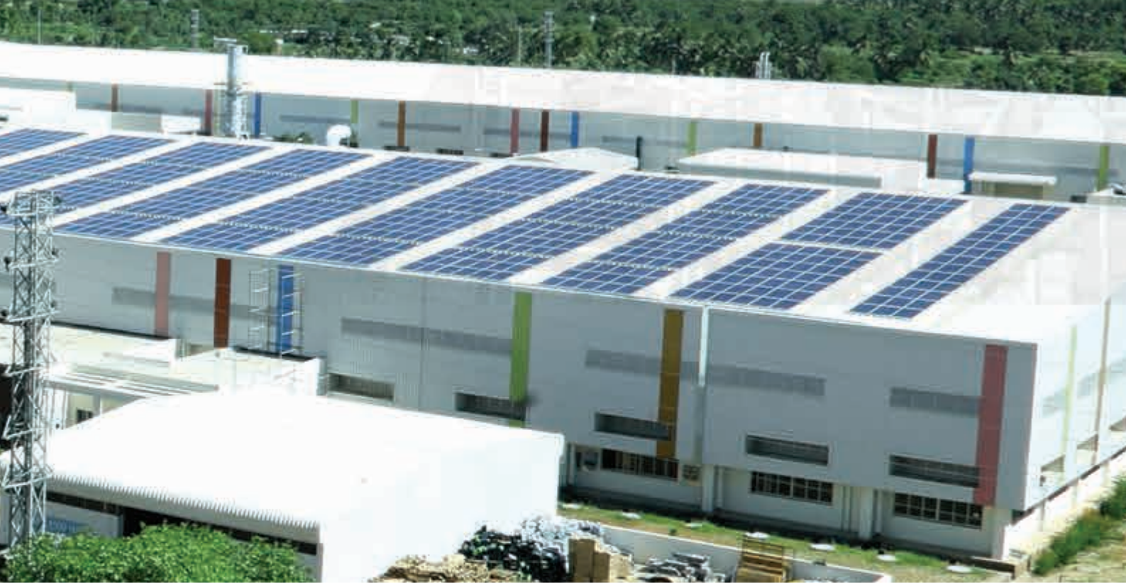
MVRLA plant at Nunegundlapalle Village, Chittoor District with Solar Roof Tops.
