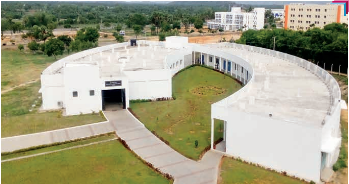
Aerial view of the Amara Raja Skill Development Center
