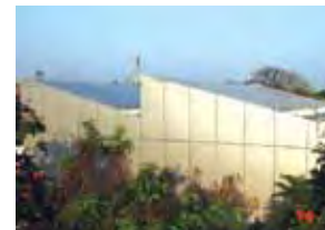
22.4kWp Solar installation at Numeric's Puducherry Plant
